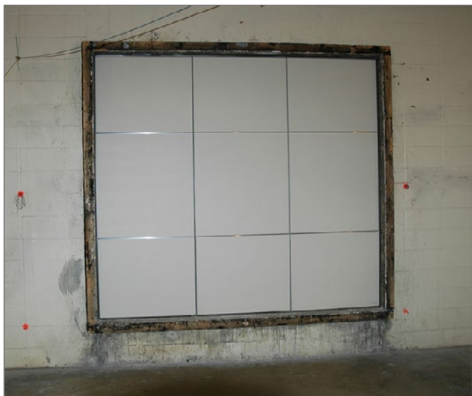
Figure 3: DIRTT walls installed to fill chamber to chamber opening.
